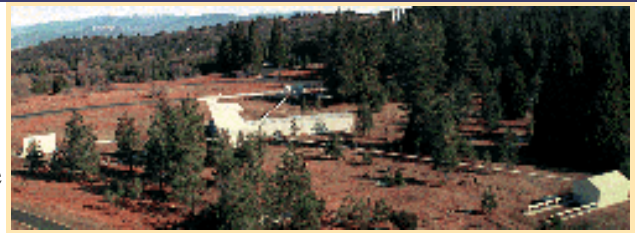
An aerial view of the Palomar Testbed Interferometer , funded by NASA to demonstrate technology for ground-based interferometry. Light collected by three small telescopes in the three small buildings is directed through pipes to the central beam combining building. The separation among the three telescopes is 110 meters.
