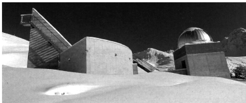
Figure 3. The François-Xavier Bagnoud Observatory. The building itself is a summary of the history of astronomy, with the oldest astronomical instrument at the North (the large triangle aligned with the meridian serves as gnomon for a big sundial), and the most recent ones at the South (the dome houses a 60-cm telescope equipped with a CCD camera).
